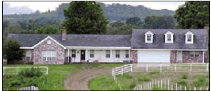
OWNER WANTS AN OFFER ON THIS HORSE LOVERS DREAM: This 120 acre ranch is at the end of a private lane w/improved pasture divided into 6 fenced areas w/live water in each. Barns & outbldgs are in place w/a professional dog kennel w/concrete slabs, electricity & water. A 4000+ SF home framed by a backdrop of mountains in the dist. 2 FP's, 2 liv areas, one w/wet bar & many built-ins, 2 utility rms, 2 MBRs, office, formal DR round out this comfortable 4BR/3BA. #102707.
